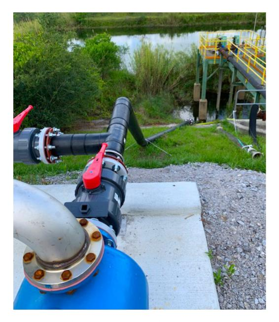
**Issue** #1 - NPSH<sub>A</sub> is  $\approx$  6.5 feet. NPSH<sub>R</sub> at BEP is 14.6 feet. NPSH<sub>A</sub> must always be more than NPSH<sub>R</sub> with as much margin as possible.
