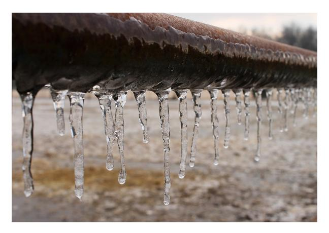
If you or your customers have a pump (and piping) that is not protected from freezing, you need to remove the water or the casing will crack and suffer expensive and permanent damage in the process. If you can't remove the water then take steps to move the item to a protected area, add some type of anti-freeze, or add heat trace/tape.
